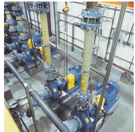
Dual pump back-up on multi-stage system. ANSI design.
